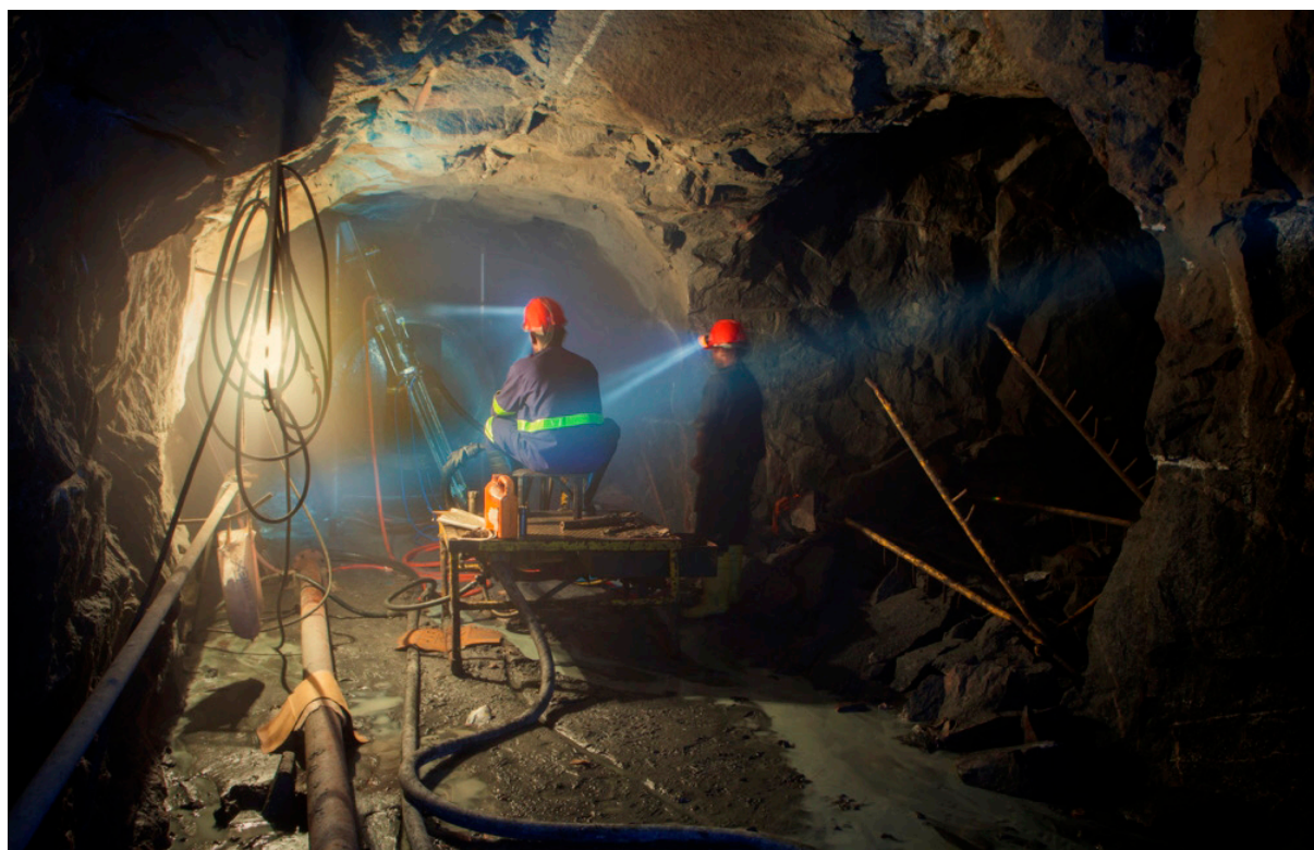
Underground drilling at MGMCL
