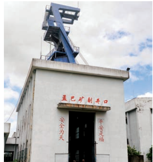
Auxiliary Shaft of BCMCL
