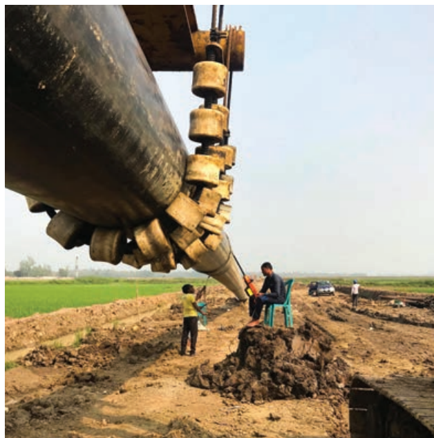
Construction Work of Dhanua-Nalka Pipeline Project of GTCL
