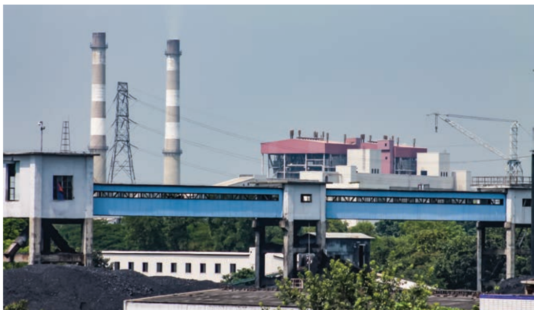
Coal conveyor belt of BCMCL
