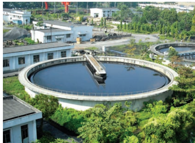
Water treatment plant of BCMCL
